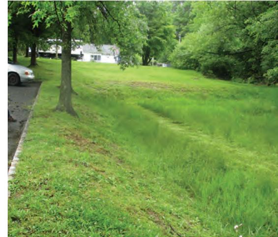
A rain garden can be installed to reduce the flooding that occurs east of the parking lot. Pervious pavement can be installed in the parking lot row directly west of the building to capture stormwater runoff from both the parking lot and the rooftop. A preliminary soil assessment suggests that more soil testing would be required before determining the soil's suitability for green infrastructure.
