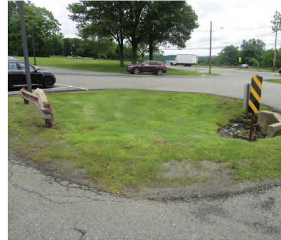
Pervious pavement can be installed in the southernmost row of the parking lot to capture, treat, and infiltrate stormwater runoff from the parking lot. A preliminary soil assessment suggests that the soils have suitable drainage characteristics for green infrastructure
