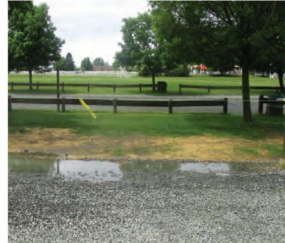
A rain garden can be installed along the northern edge of the parking lot area to help infiltrate the pooling stormwater in that area. A preliminary soil assessment suggests that the soils have suitable drainage characteristics for green infrastructure.
